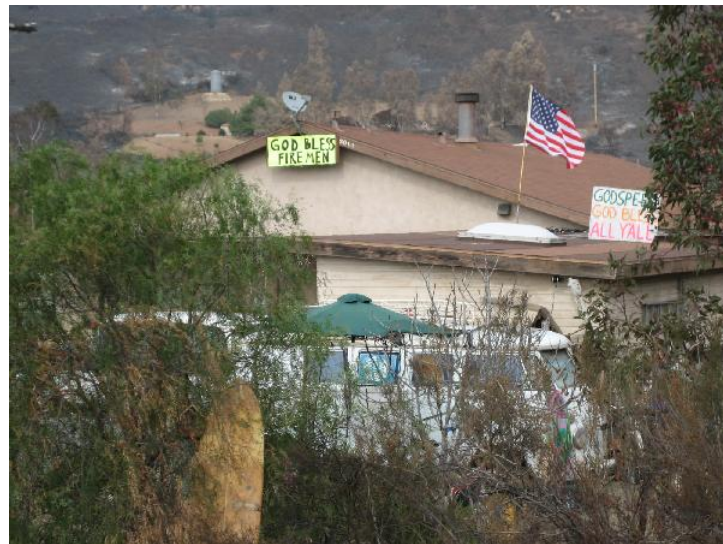
This house was saved while all the homes around it were burned to the ground.
